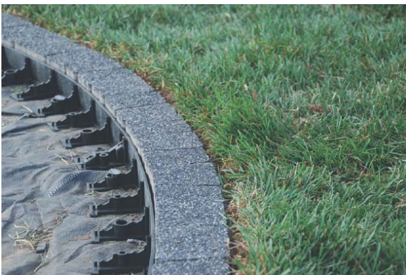
The final phase of Garden Edge Pro borders installation is to cover them with soil, grit, bark, etc., so as to make them invisible.
